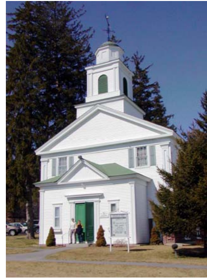
52 Main Street Center Harbor, New Hampshire
